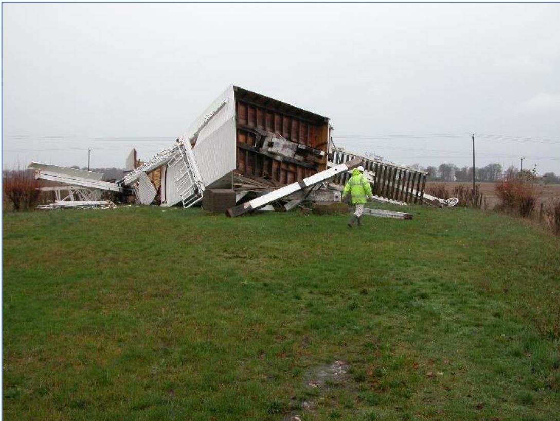
Figure 5 Chillenden windmill, blown down in 2003, now re-built
